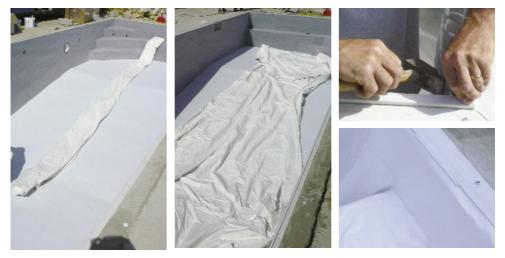
Take the liner out and unfold it lengthways. Traces of creases may remain on the liner once it has been removed from its packaging (particularly on dark colours). This is completely normal and will disappear after a few days, once the pool has been fully filled with water, and subject to normal conditions of use and treatment (water temperature and balance).
