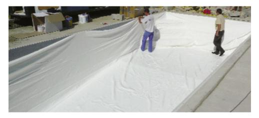
• Then position the step unit so that the welding between the bottom and the step unit coincides with the edge of the last riser. Centre the step unit and lift the material towards the top. The pressure of the water will always tend to drag the step unit down.
