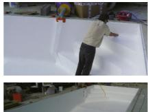
last wrinkles by pushing the bottom towards the walls and place the corners in their fi nal position. The liner must be stretched evenly without any pulling. There should be no creases on the bottom when the pool is filled.
